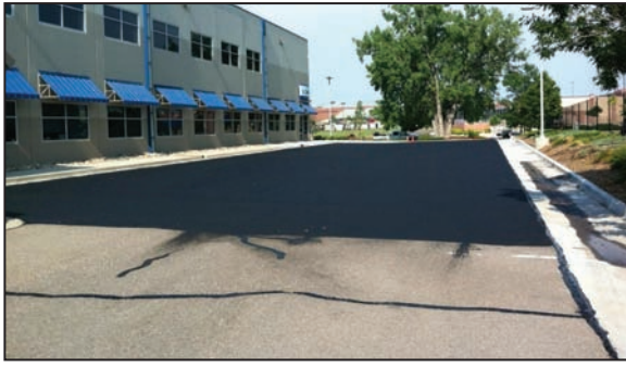
Pitch Black Seal-coat transforms a lot.
